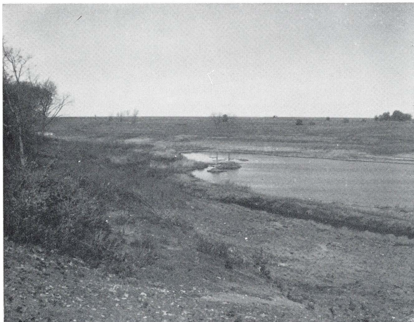
A scene from a newly completed dam in the Frog Creek Watershed District.
